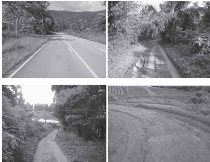
Figure 4. Various road conditions measured in this study.
