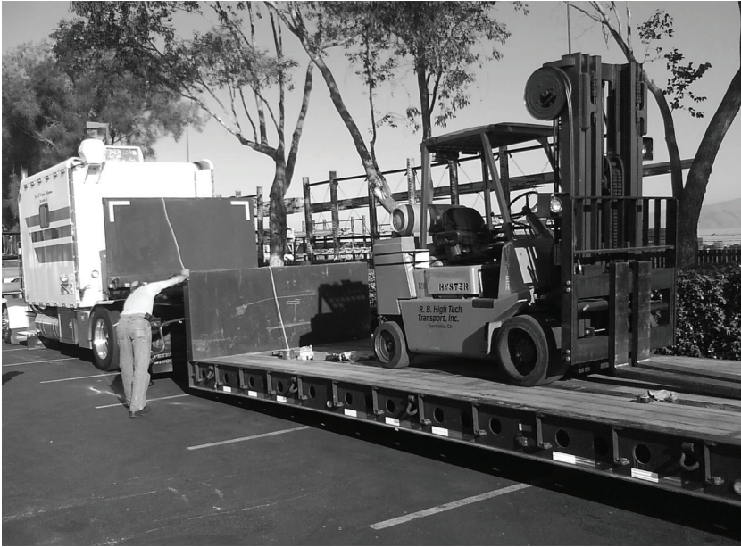
Figure 2. A 12-ton forklift used as a substitute mass for the test move.
